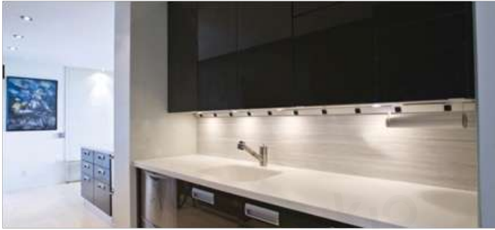
Figure 142. Undercabinet lighting illuminates preparation areas in the kitchen and hence is a task lighting
