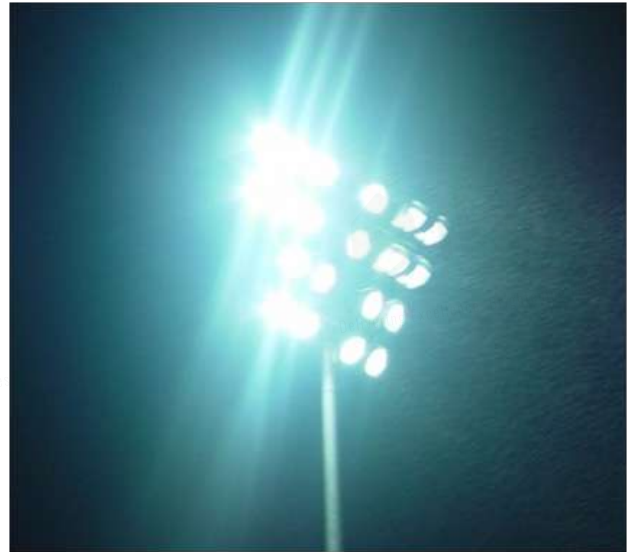
Figure 134. Glare from sports lighting in a stadium
