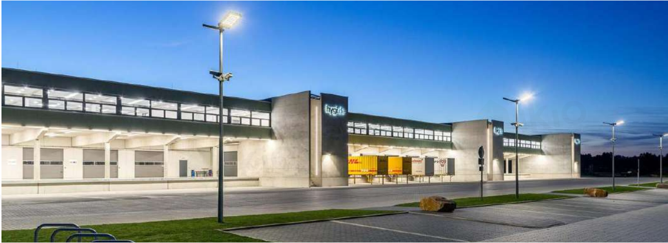
Figure 57. Area Luminaires in a parking lot
