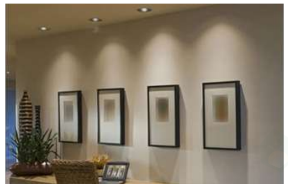
Figure 141. Accent lighting focussed on paintings
