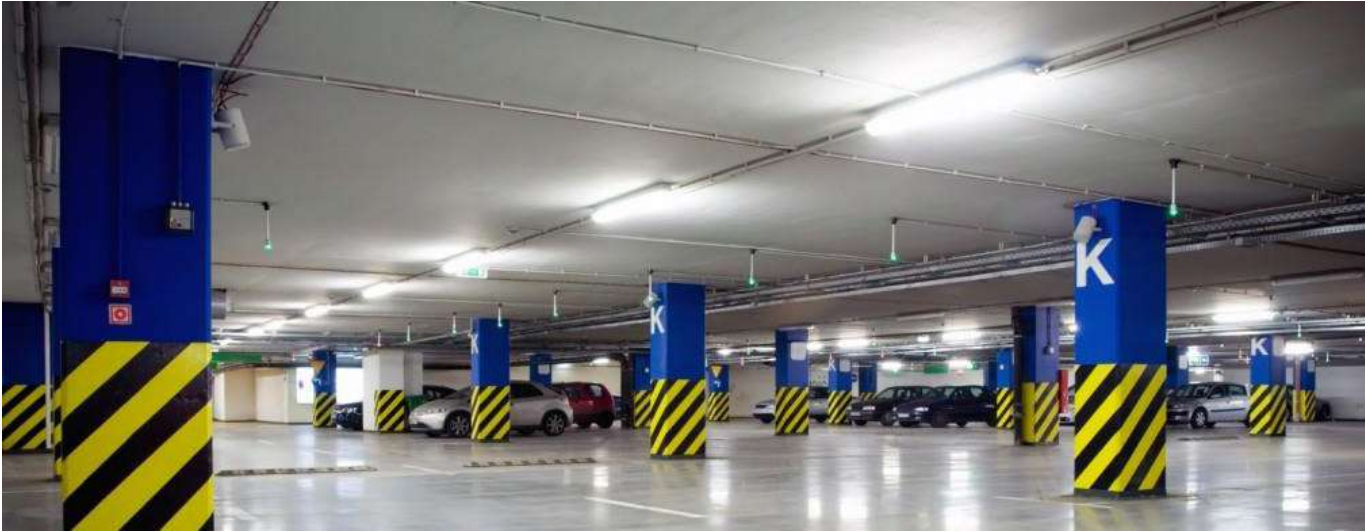
Figure 79. Tri-proof luminaires are vandal resistant and see major use in underground parking areas
