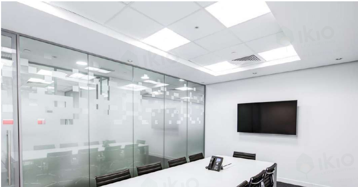
Figure 83. LED Panel lights are widely used in office settings because of their low profile designs
