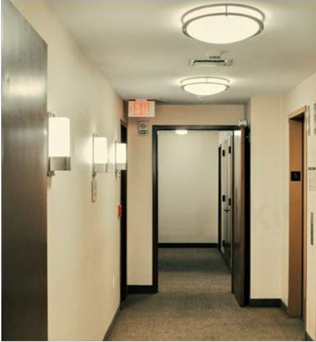
Figure 94. A hallway with flush mount lighting and sconce lighting
